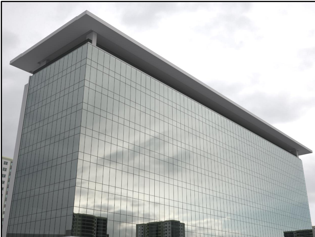
SGG CLEAR COSMOS UNDER OVERCAST CONDITIONS
